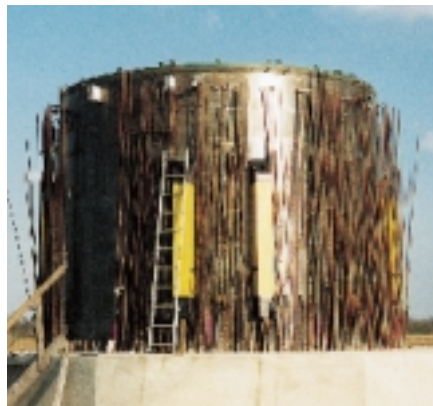
Interior formwork for base section
