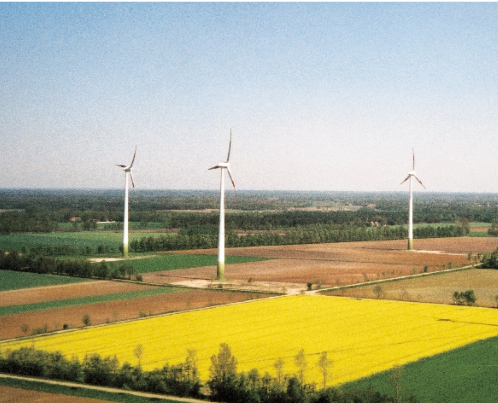
One of two windparks in Meppen, Germany, with 6 windmill towers each, hub height 98 m
