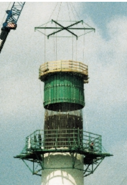
Exterior formwork is lifted in place
